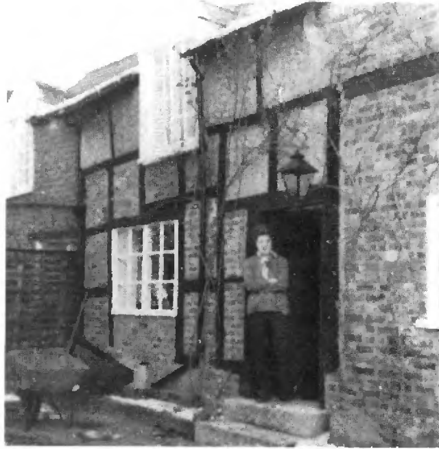
Passage between kitchen and former dairy
