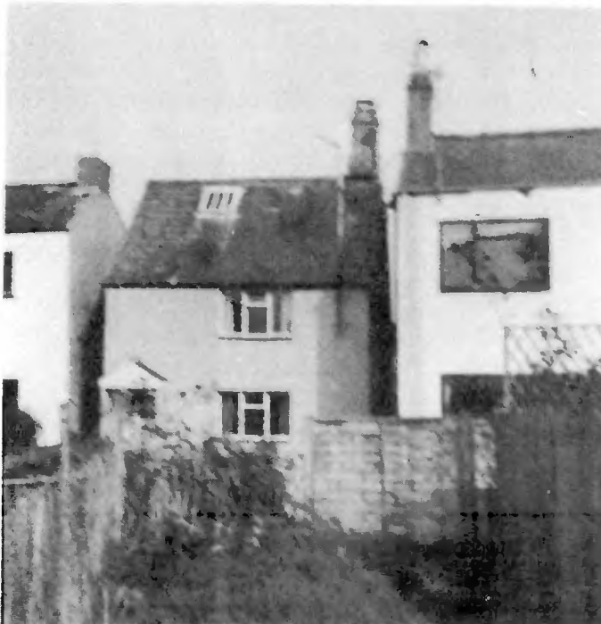
No. 49 from West - i.e. from the footpath.
