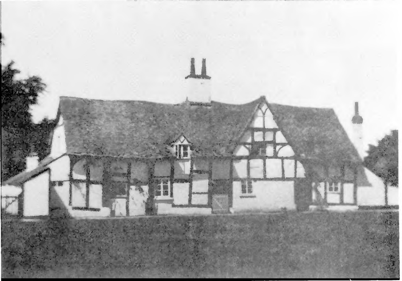
The Home Farm, shortly before demolition. Photograph lent by Mr Mitchell
