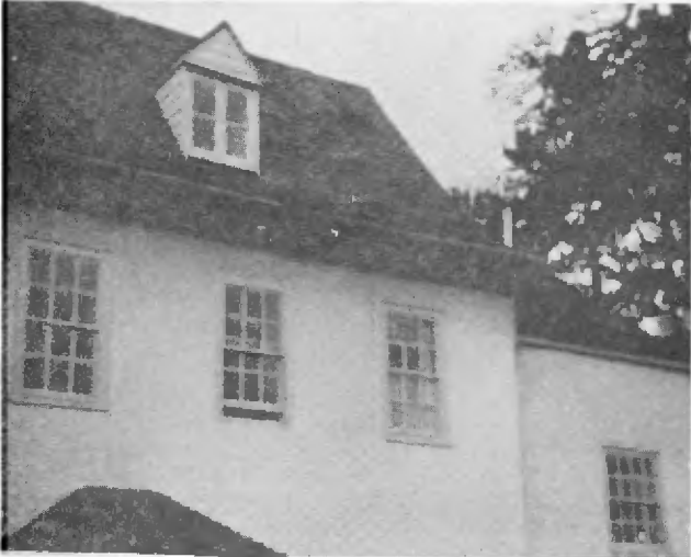
A new four-pane window for the small chamber over the former "guilt" room.
