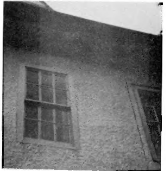
A three-pane window without a sill, woodwork flush with brickwork
