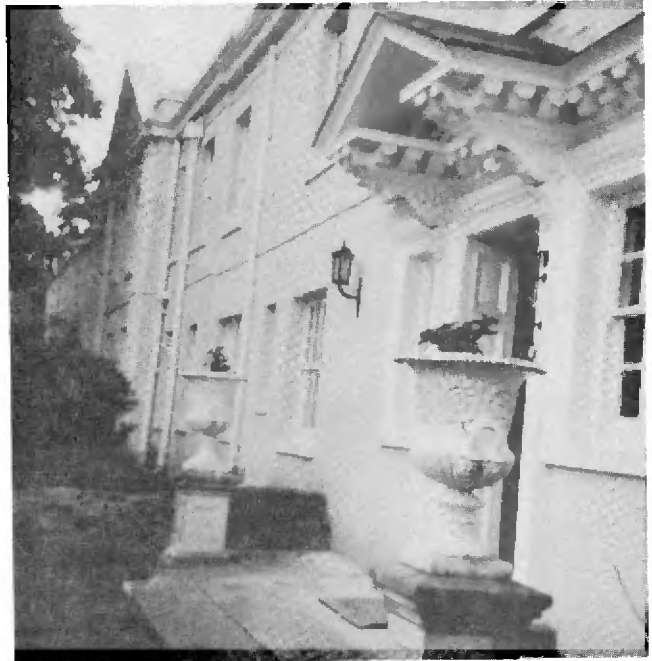
Drive front and entrance
