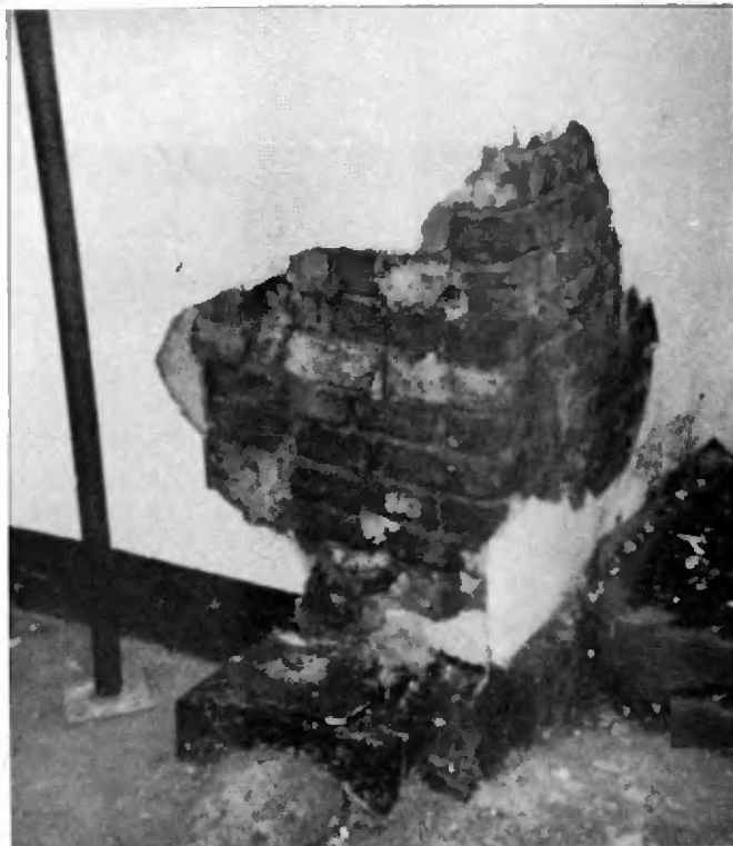
No stone foundation east of present front door.
