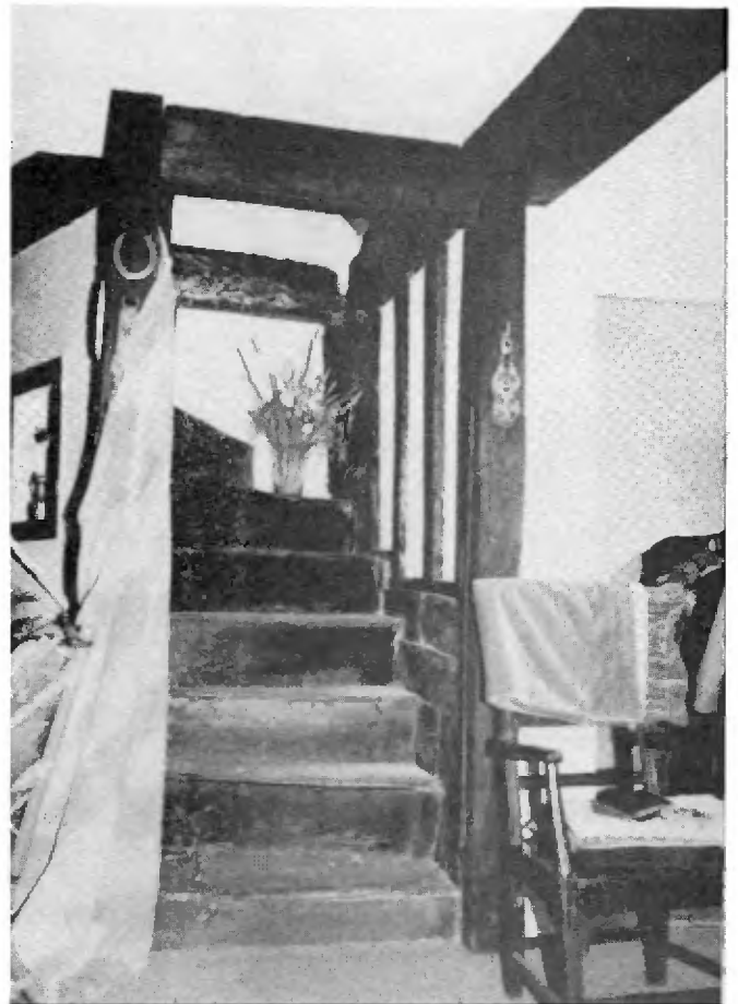
The winder stair and close-studding
