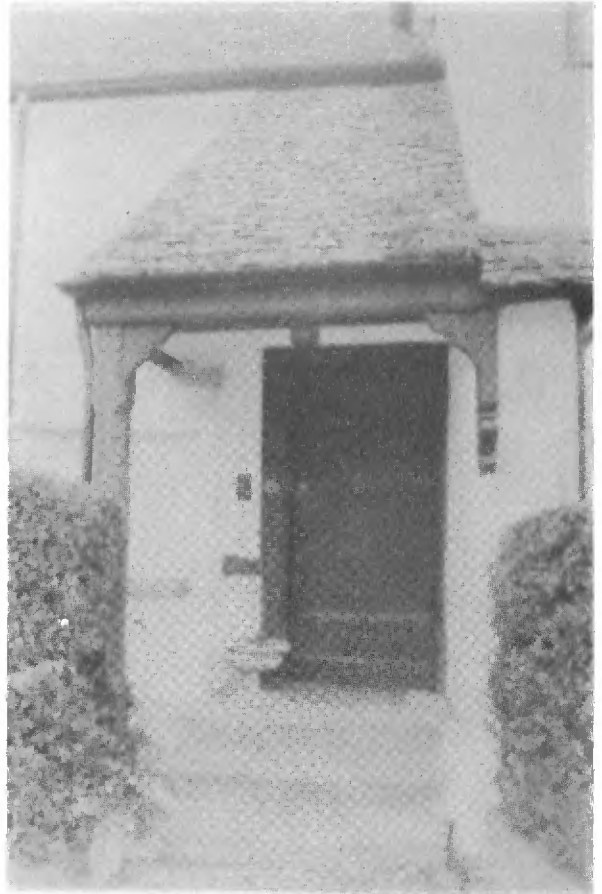
The porch and front door
