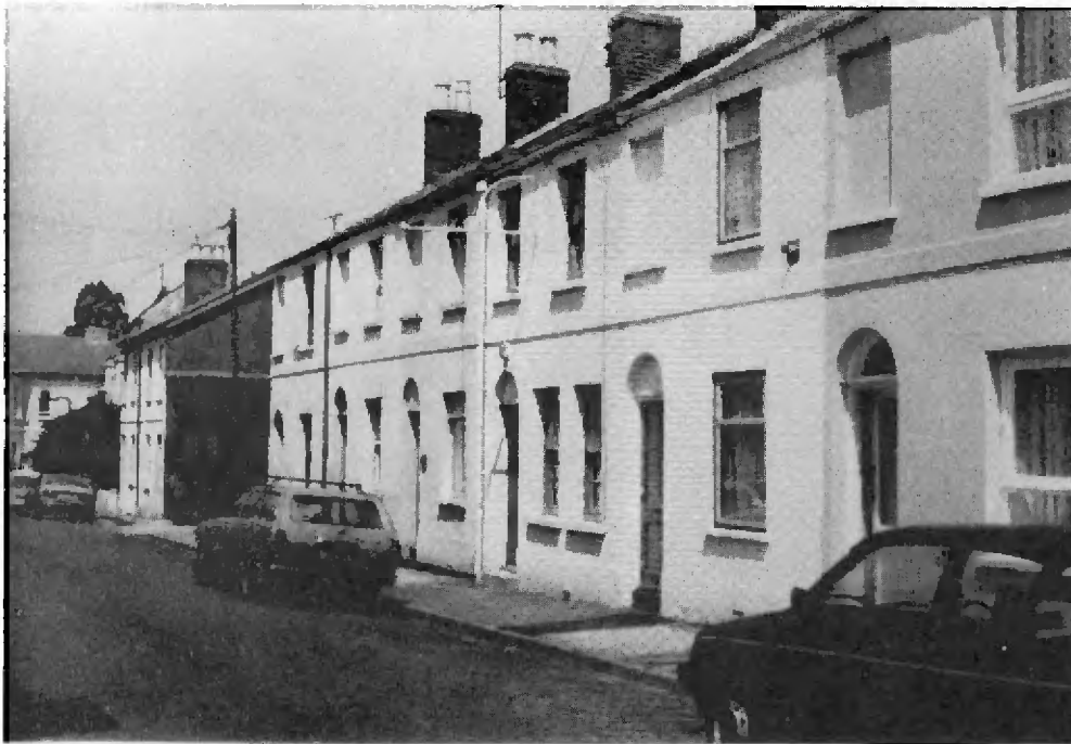
2. The north side of Rosehill Street, showing Nos. 6-8 and 18-28. The metal bracket which once held an inn sign may be seen on No. 24, formerly the 'Black Horse Inn'.
