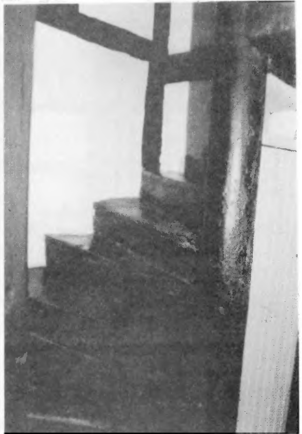
Stairs to first floor
