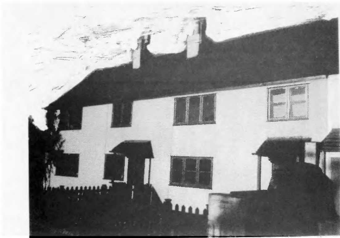
As they are - new windows, doors, and porches
