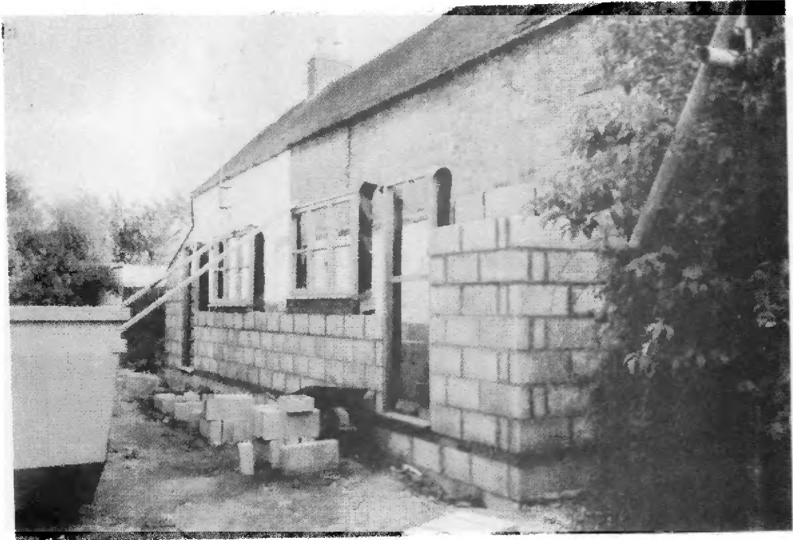
Building work at the back
