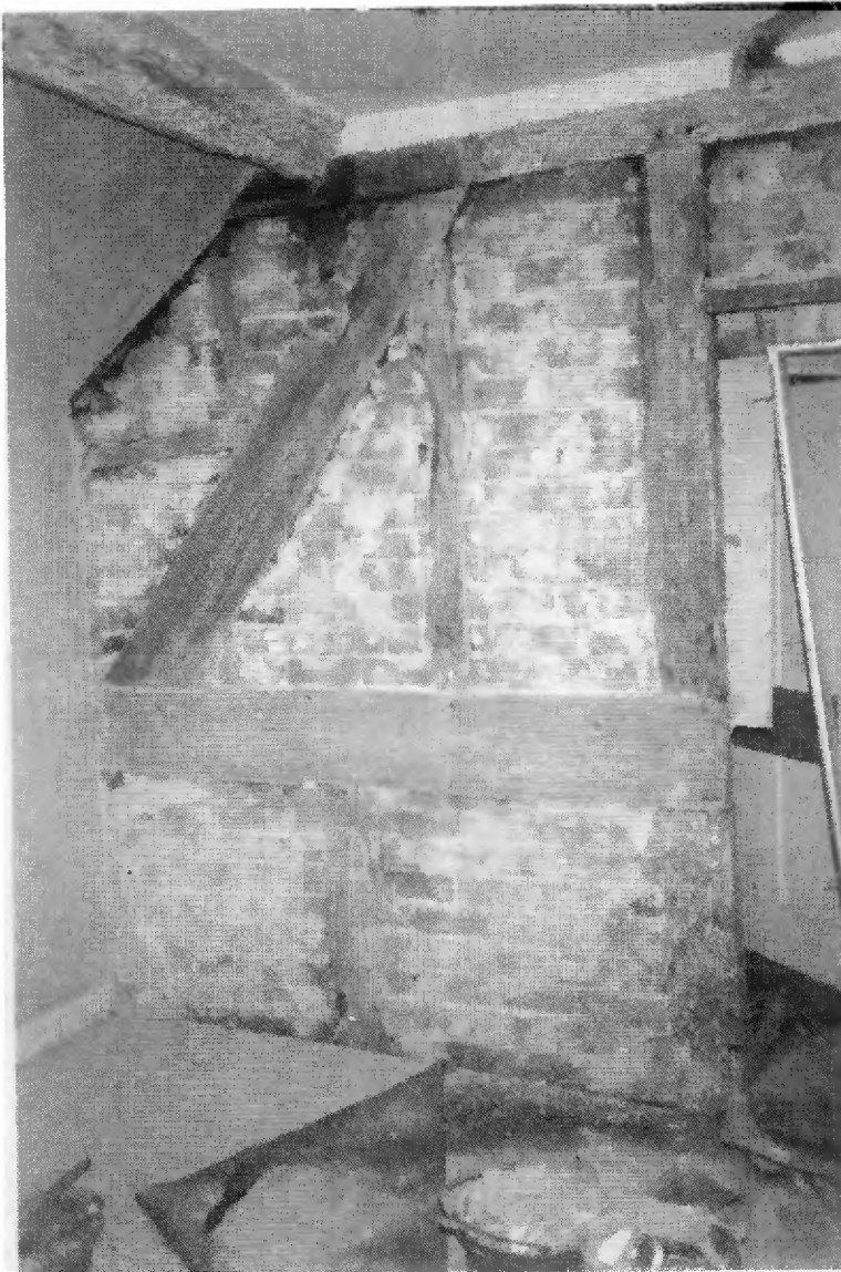
Timbers uncovered during the restoration
