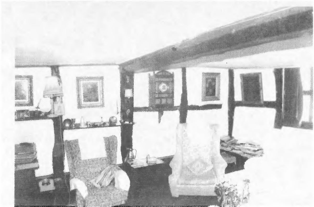
Parlour - timber framed east wall
