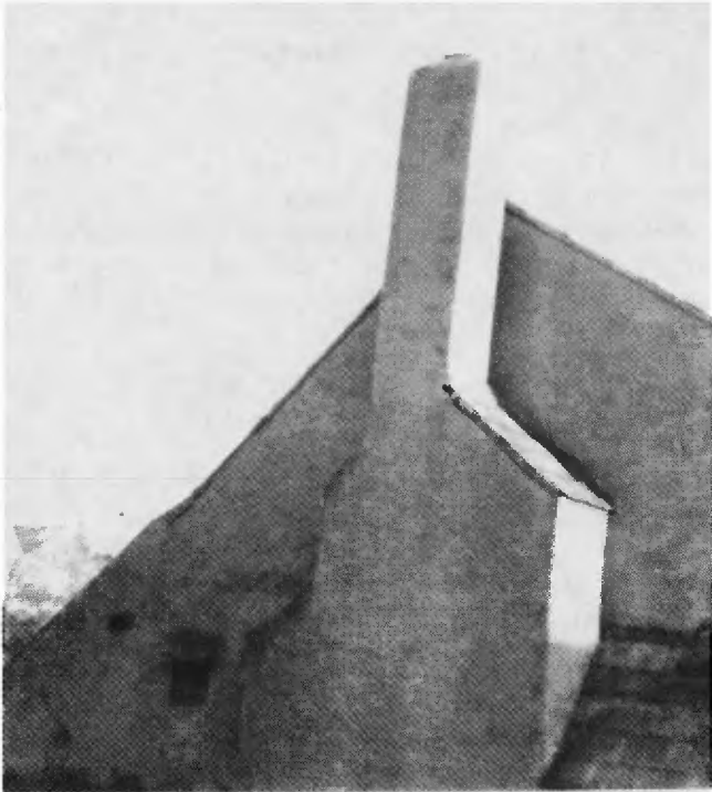
Detached chimney at west end of house
