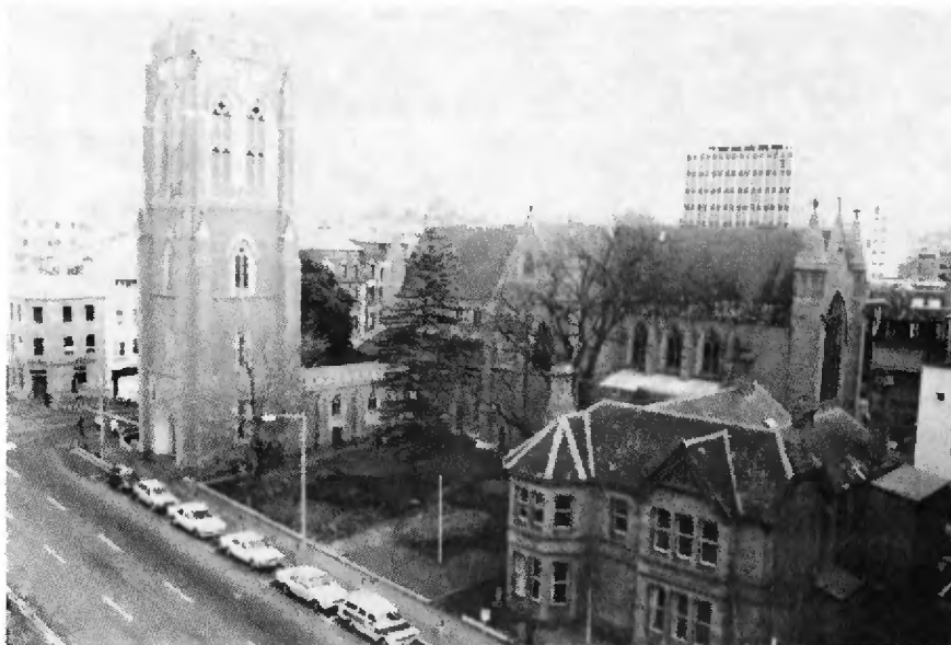
The former Deanery, now Offices.
