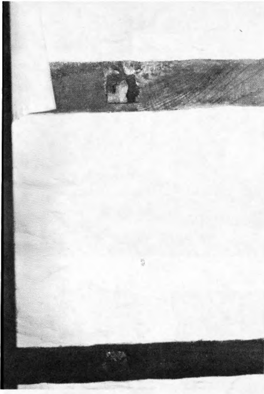
Cheese-room - holes in horizontal timbers to take brackets to support shelves. (L.H.)
