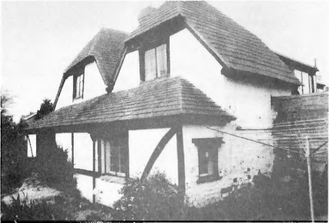
3. South end, showing dairy wing and modern single-storey extensions.
