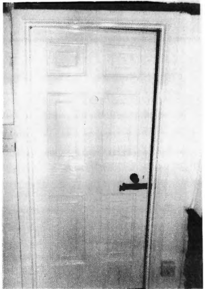
18. Parlour door, seen from the entrance hall. Early 19th century panelled door
