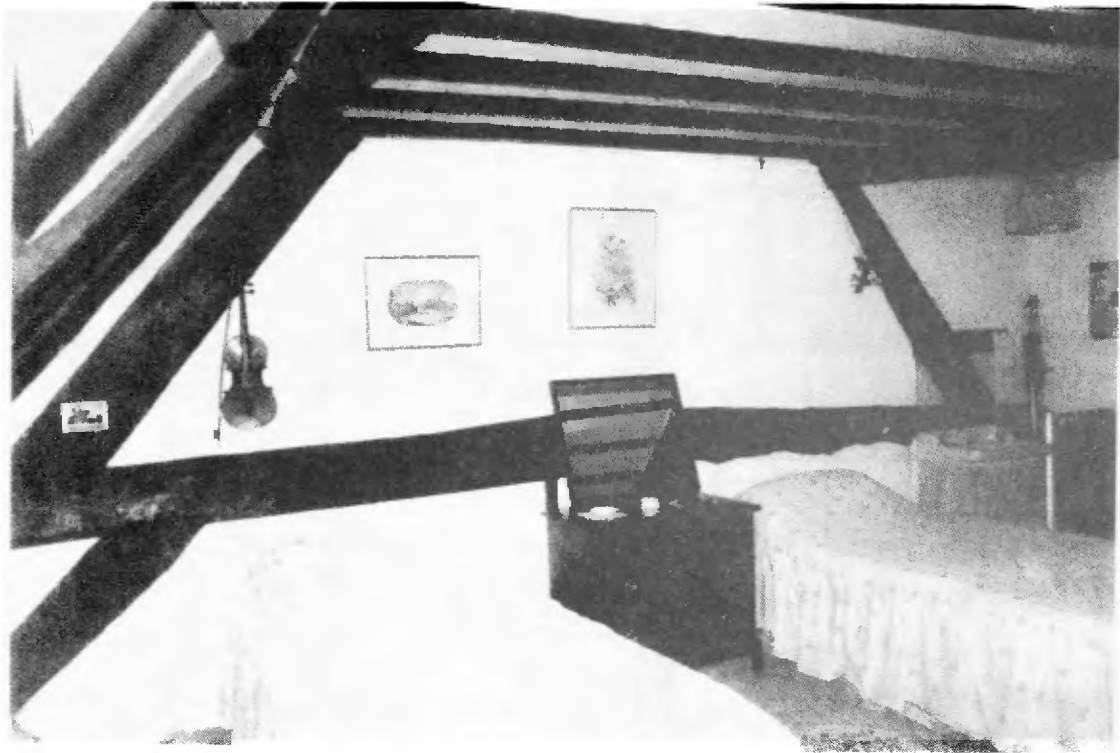
15. Truss 2, viewed from the south
