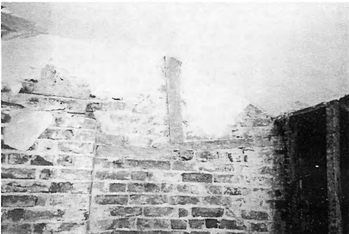
Parlour chamber - East wall rebuilt and timbering inserted haphazard
