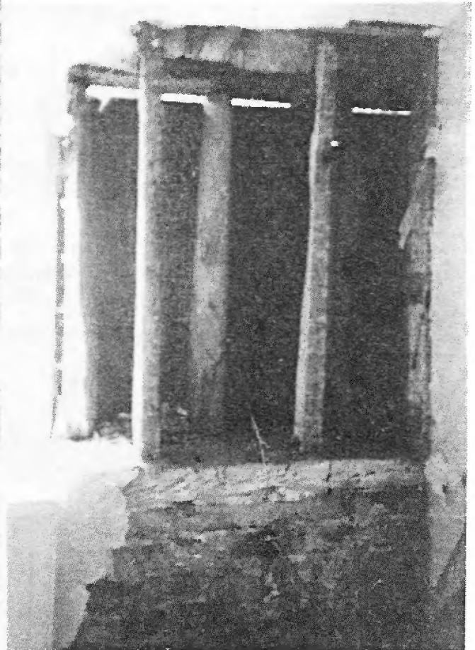
Wall plate and double timbering, middle room
