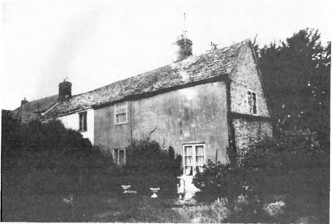
North half of the house (No 1)
