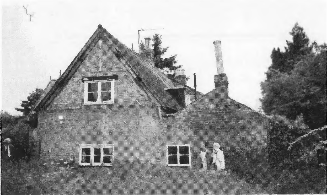
Northern end of building
