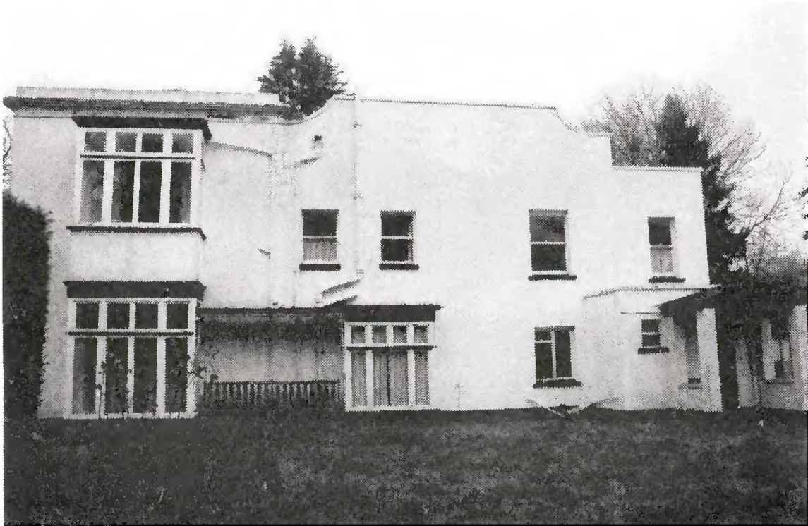
Secondary Entrance on Right Hand Side Added When House Divided into Two Dwellings
