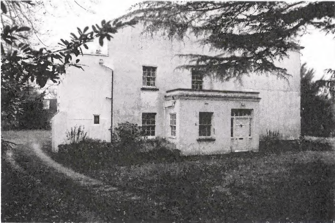
Main Entrance on Left Hand Side
