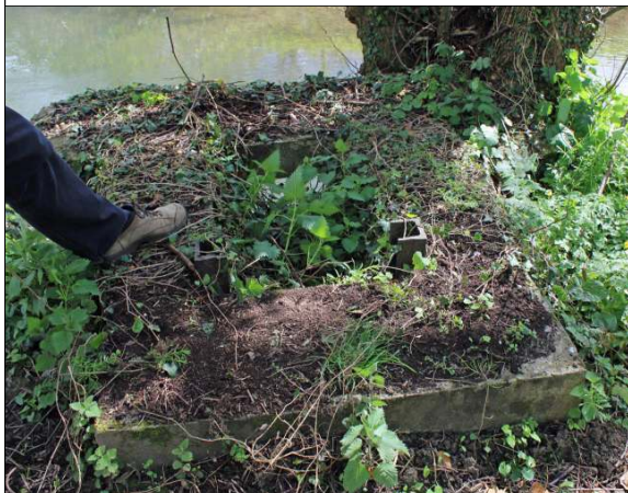
Probable inlet for water from the River Frome at the eastern end of the plantation. Pair of iron channel pieces still in place which would have carried a stop board some 2 feet wide. Some form of pump was probably necessary to lift the water from the Frome at this location.
