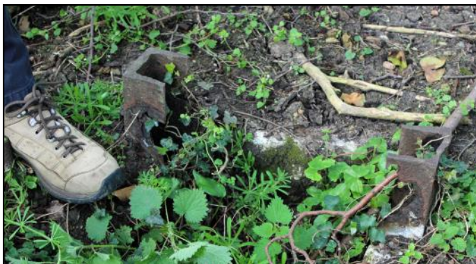
Figure 3: A pair of iron channel pieces still in place (in April 2014) which would have carried stop boards.
