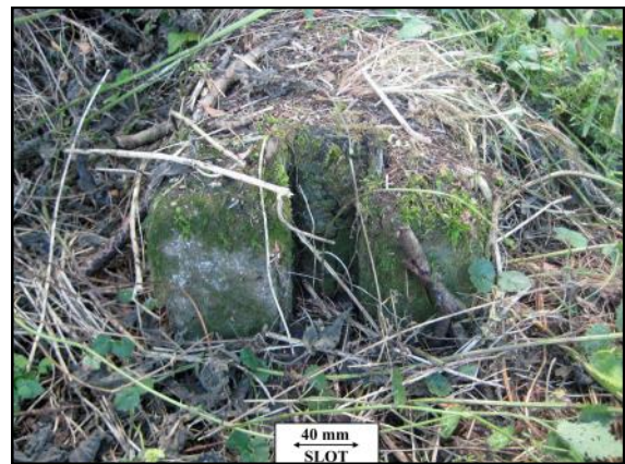
Figure 2: A close up showing the remains of one of the water channels and the slot for a control board. U-shaped iron channels were set into each slot to allow the boards to be adjusted easily. A few remain in situ. Most were probably removed for scrap many years ago.
