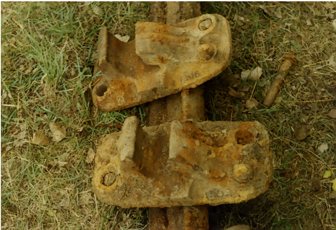
15-foot rails and 1896 dated chairs which once supported a stop block, unearthed from the end of the embankment.
