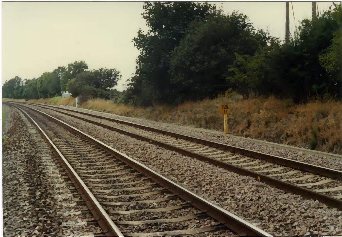
The Gloucester - Bristol main line looking west at the site of the junction for Gossington sidings. The points were situated on the extreme right of the photograph at 106 miles 39¼ chains from London Road, Derby.
