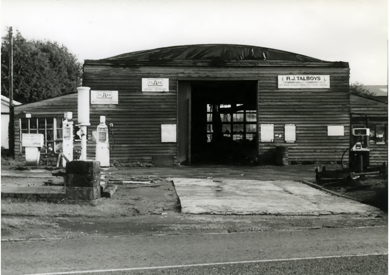
Gardiner's garage, Cambridge, Glos, built from materials recovered from Slimbridge magazine. The roof is supported on 8 Belfast roof principals. Demolished end October 1993.
