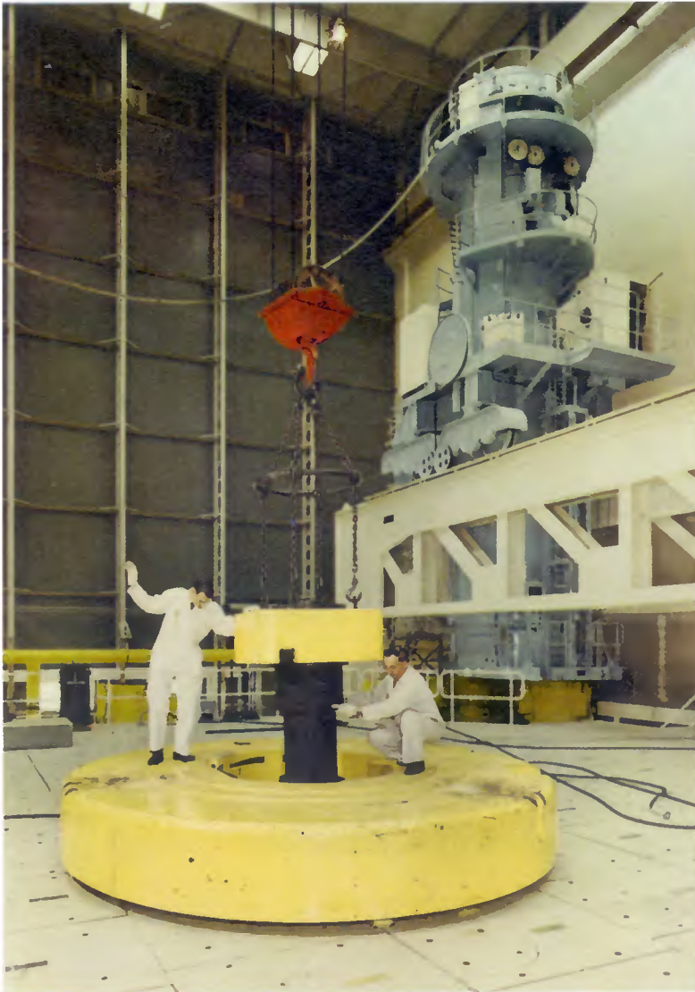
Reactor No. 2. Positioning chute headbox on standpipe
