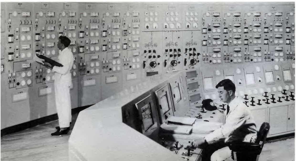
Main control room
