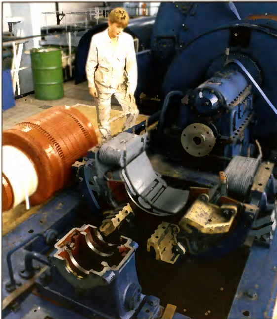
Routine maintenance on the turbo/generator exciter.
