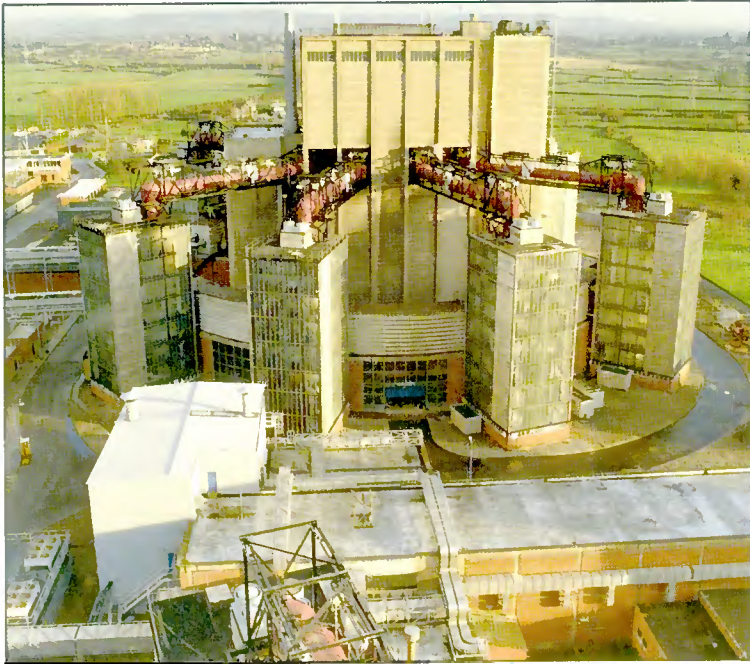
Four of the boilers which serve No. 2 reactor.
