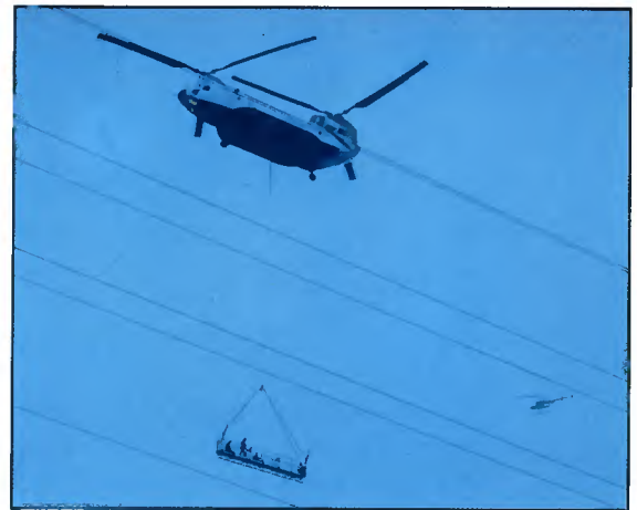
Europe's first airborne power-line repairs. A 275kv line spanning the river Usk at Newport South Wales was repaired through the use of a cradle suspended from a powerful helicopter. The CEGB saved £250,000 over conventional repairs – and the work was completed in 45 minutes rather than several weeks.
