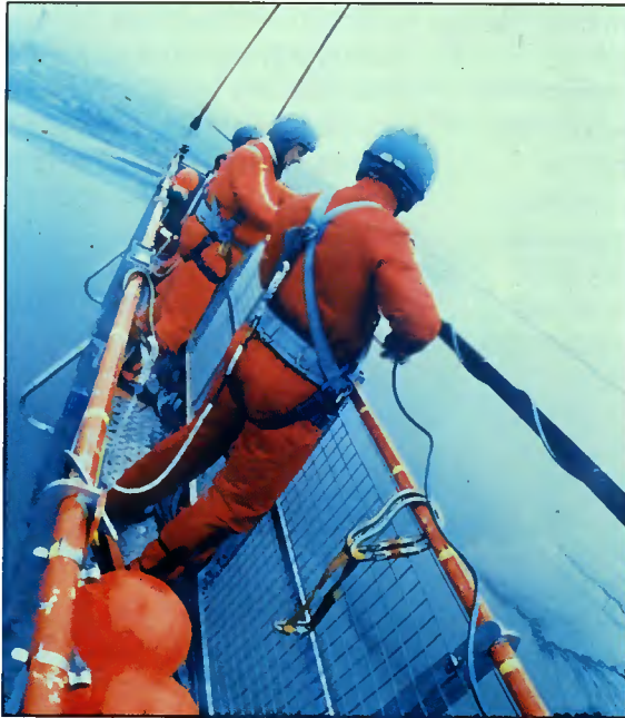
Europe's first airborne power-line repairs. A 275kv line spanning the river Usk at Newport South Wales was repaired through the use of a cradle suspended from a powerful helicopter. The CEGB saved £250,000 over conventional repairs – and the work was completed in 45 minutes rather than several weeks.
