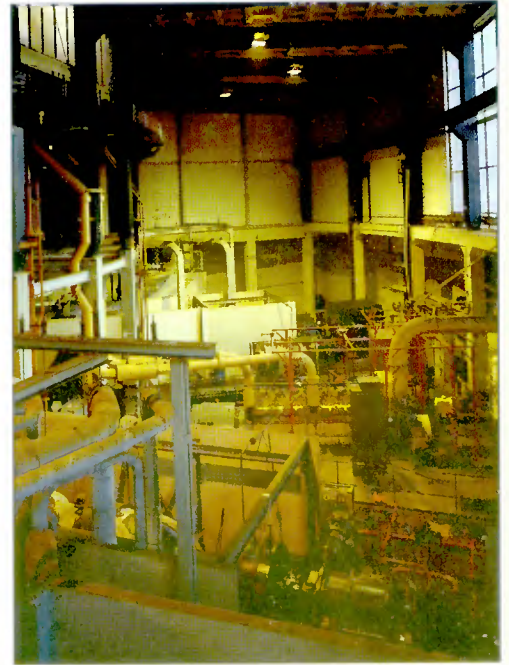
Carbon dioxide is pumped through the core by gas circulators.
