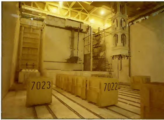
Unused element skips in an empty storage pond. A fuel transport flask can be seen behind skip 7023.
