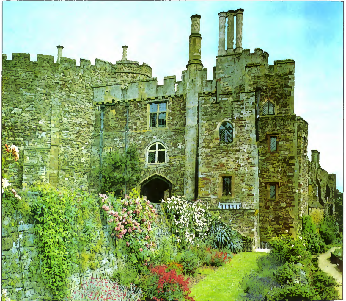
Keep and inner court entrance from the garden.
