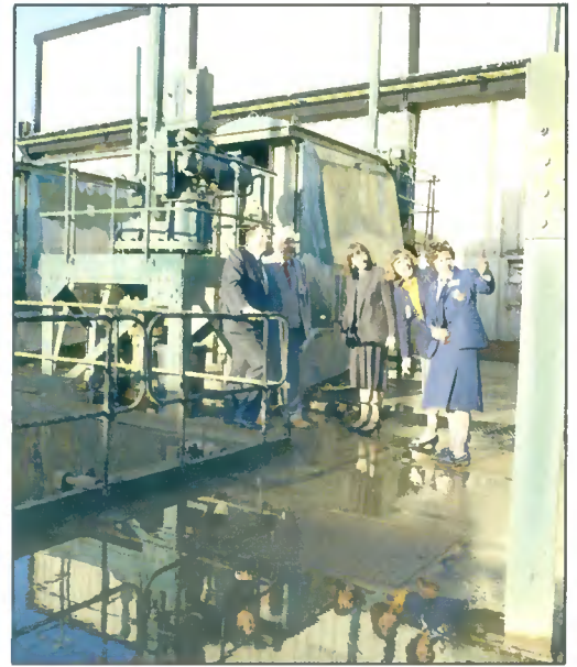
River debris is removed from the cooling water before use.
