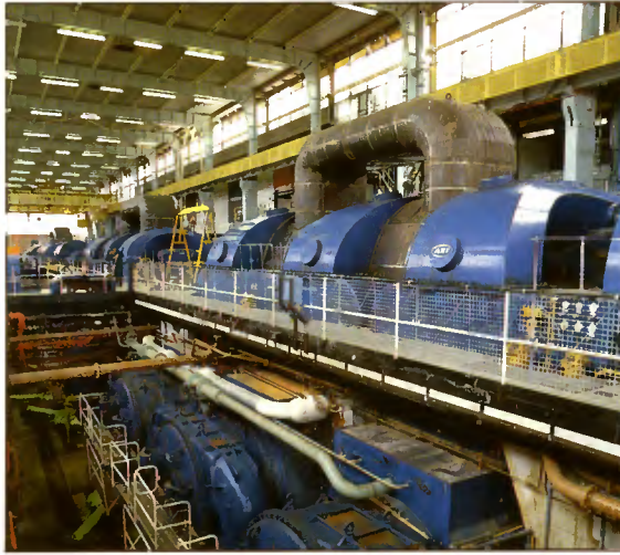
Routine maintenance on the turbo/generator exciter.
