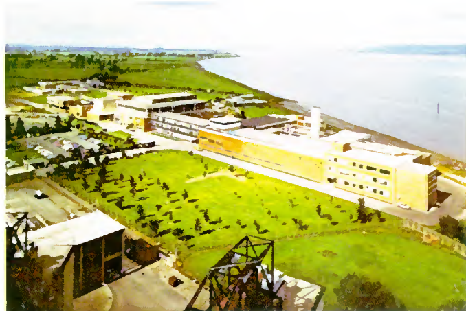
Above Berkeley Nuclear Laboratories seen from the roof of the adjacent Power Station. The Irradiated Fuel Examination Facility is nearest the camera; the white concrete cube at centre left houses the Critical Reactor Assembly. Oldbury Nuclear Power Station and the towers of Severn Bridge are visible on the horizon.
