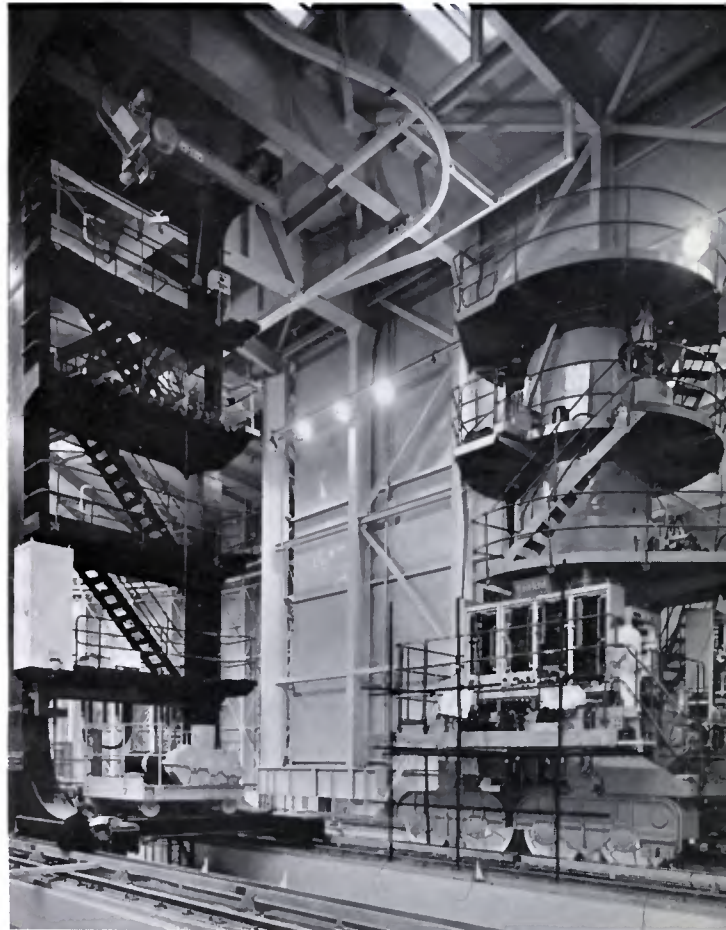
Transfer equipment and the first charge machine
