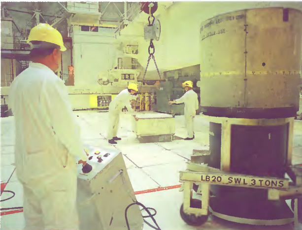
Two of the 1½ tonne floor slabs are lifted away.
