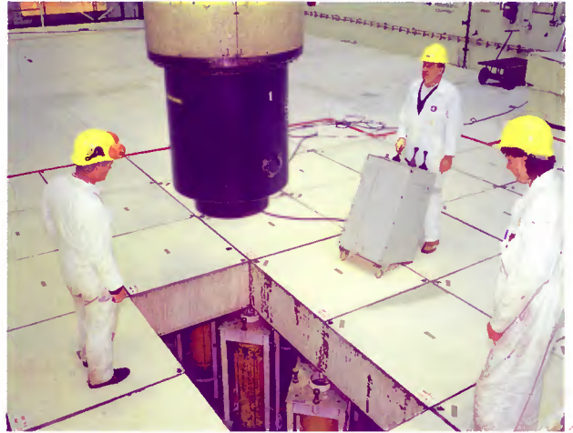
The Chute head box is lowered into place.
