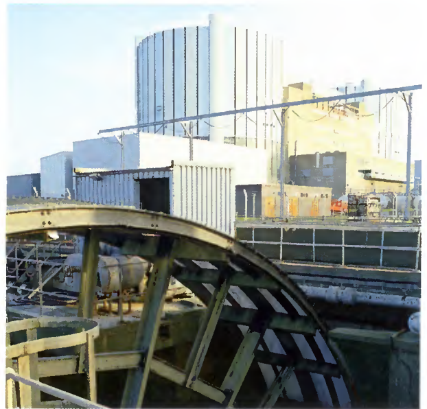
Cooling water is screened to remove debris.
