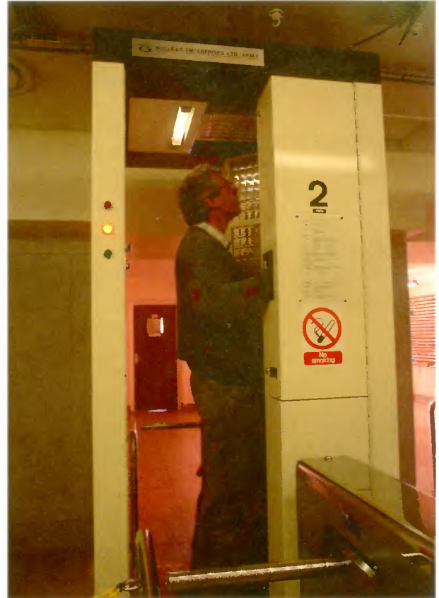
Every person must pass through a whole body monitor before leaving the reactor building.
